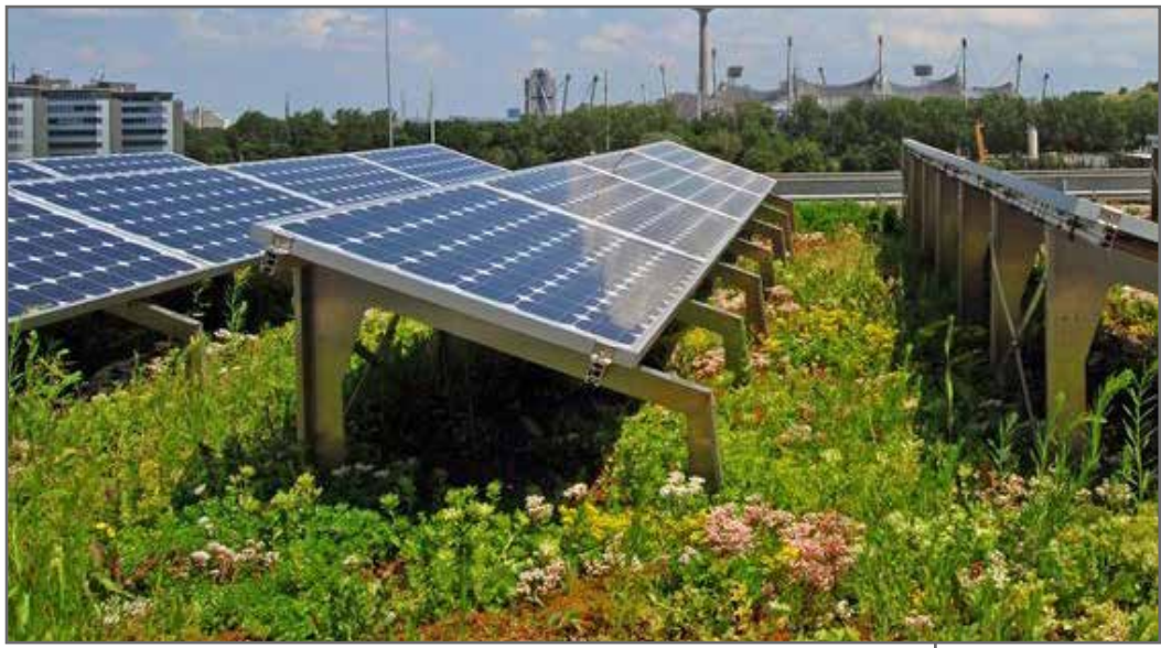
Living roof and solar pv panels
